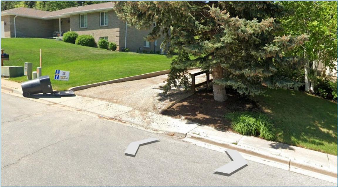
Figure 1 Gravel migration from unpaved driveway.
