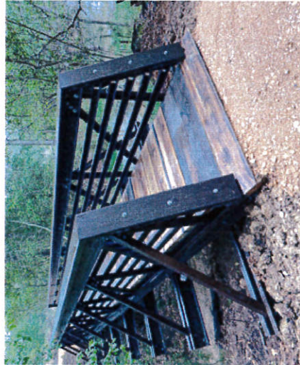
A typical pre-fab FRP bridge assembled and installed by Avid Trails.
