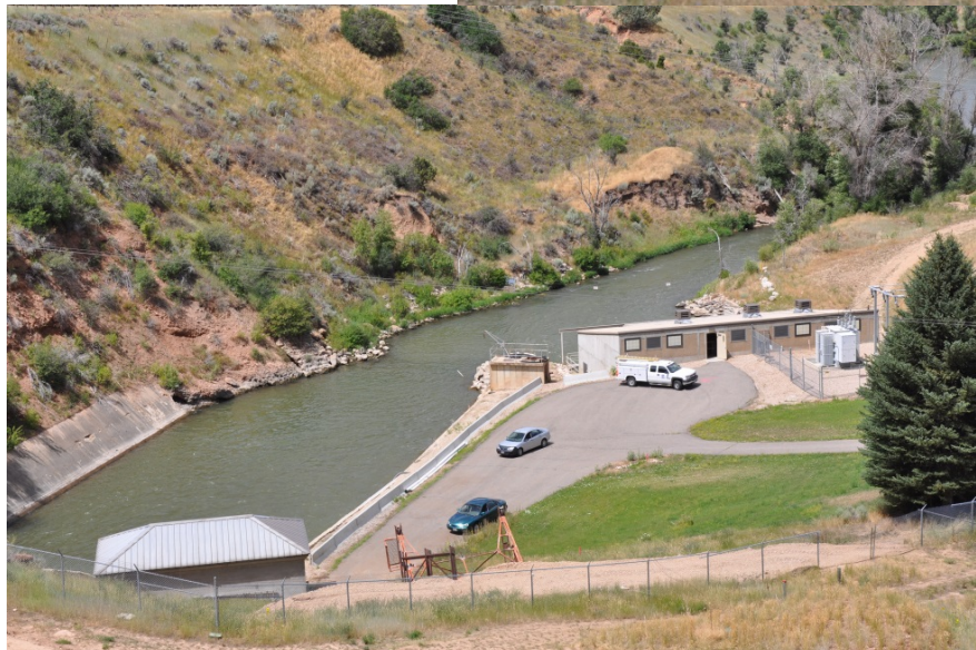
Upstream view of the plant.
