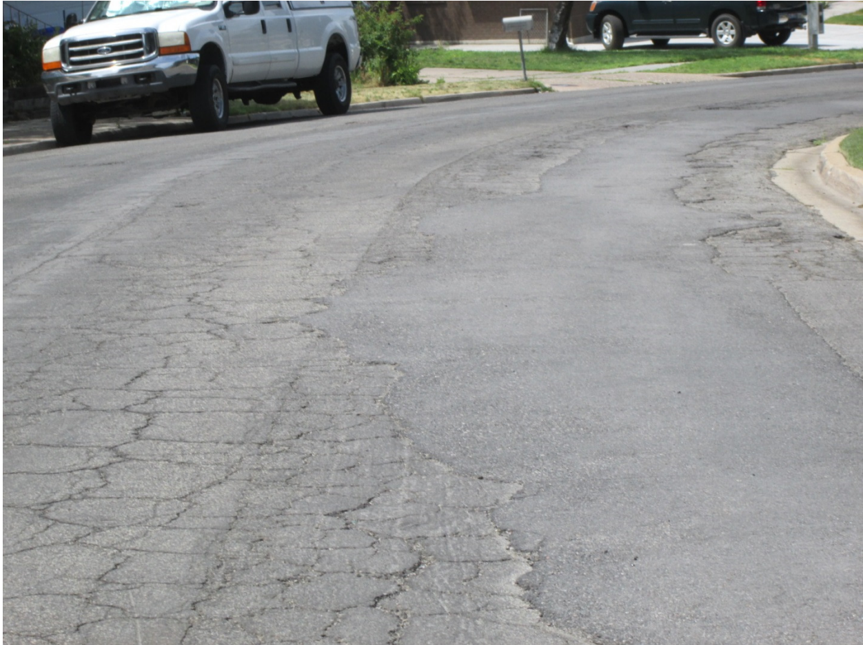
Photo 1. Poor Condition – Emerald Hills Dr from Emerald Hills Cir to Davis Blvd (RSL = 4 years)
