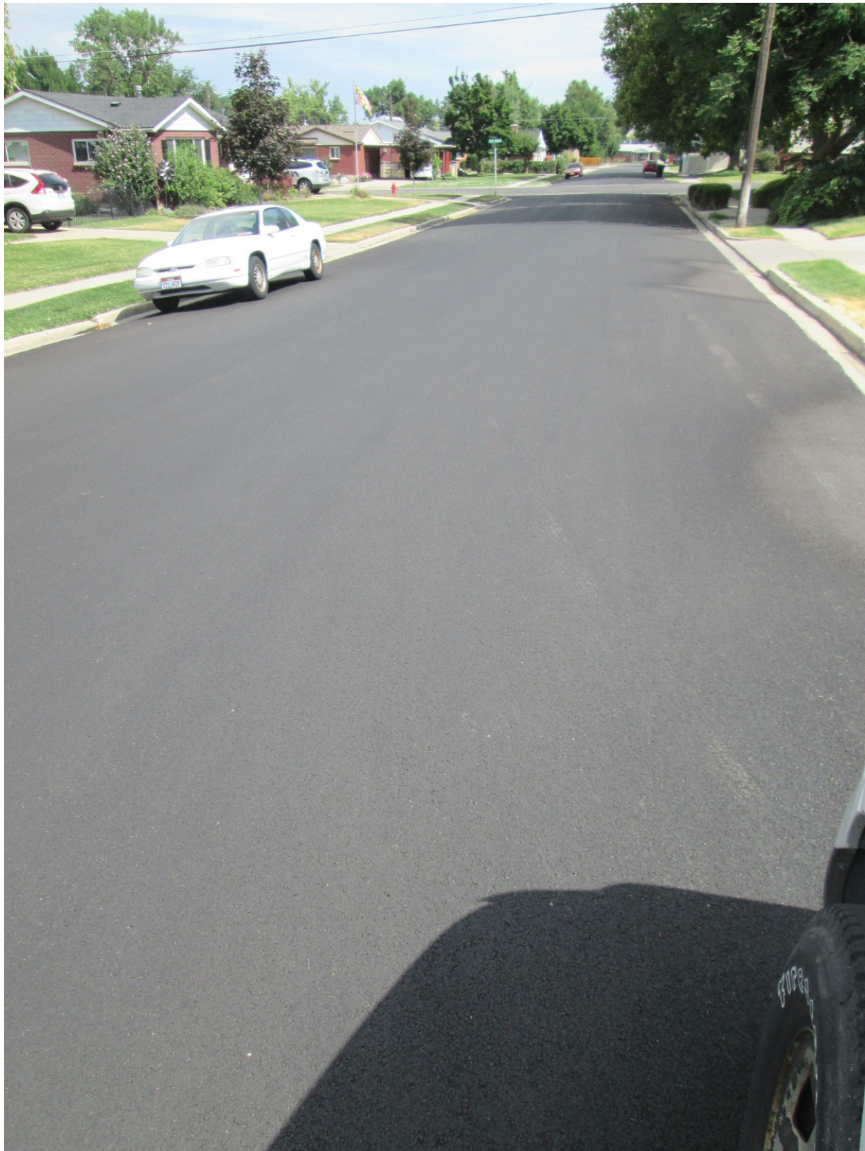
Photo 5. Excellent Condition – 200 E from 550 N to 400 N (RSL = 20 years)
