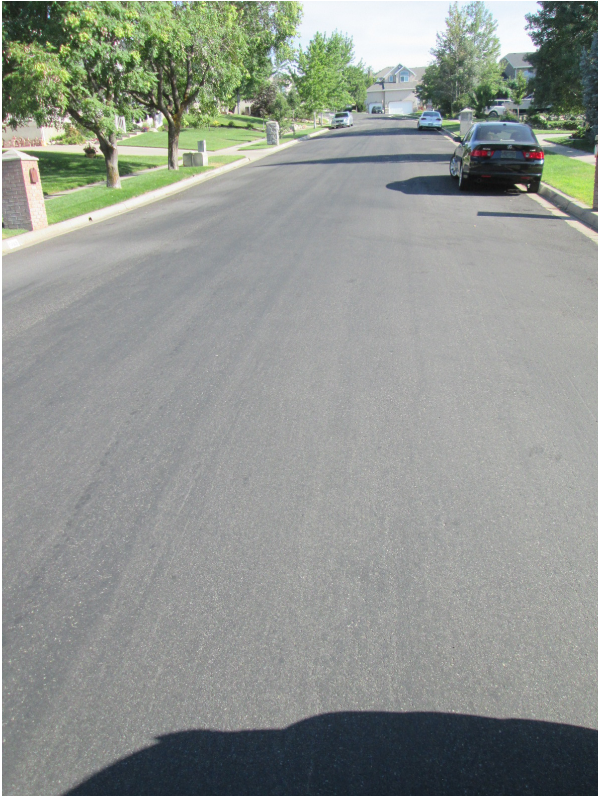
Photo 4. Very Good Condition – 250 W from Monarch Dr to City Boundary (RSL = 14 years)
