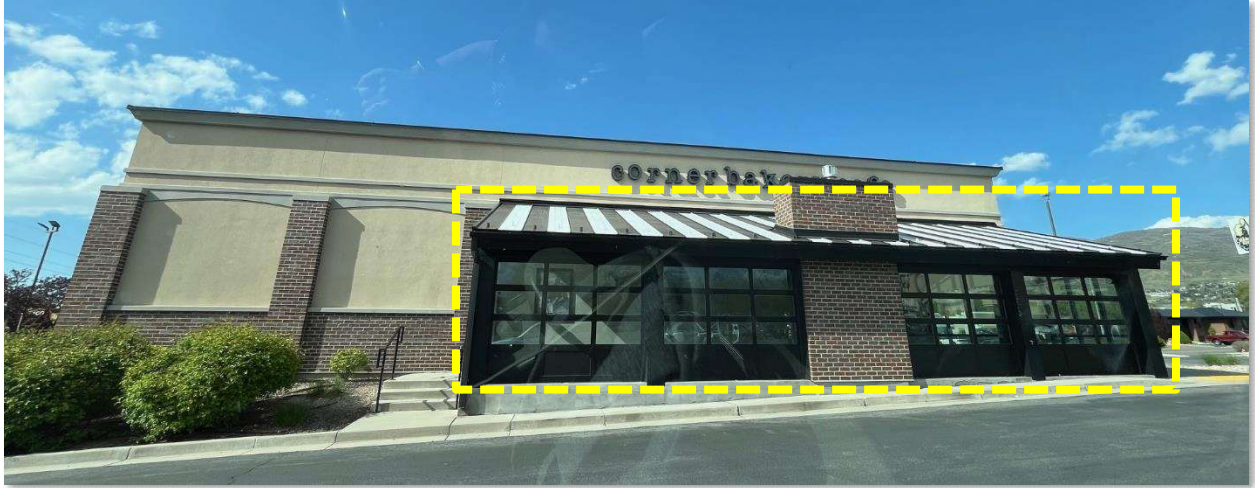
Image 1: Existing South Building Elevation – Photo Taken April 24, 2024
