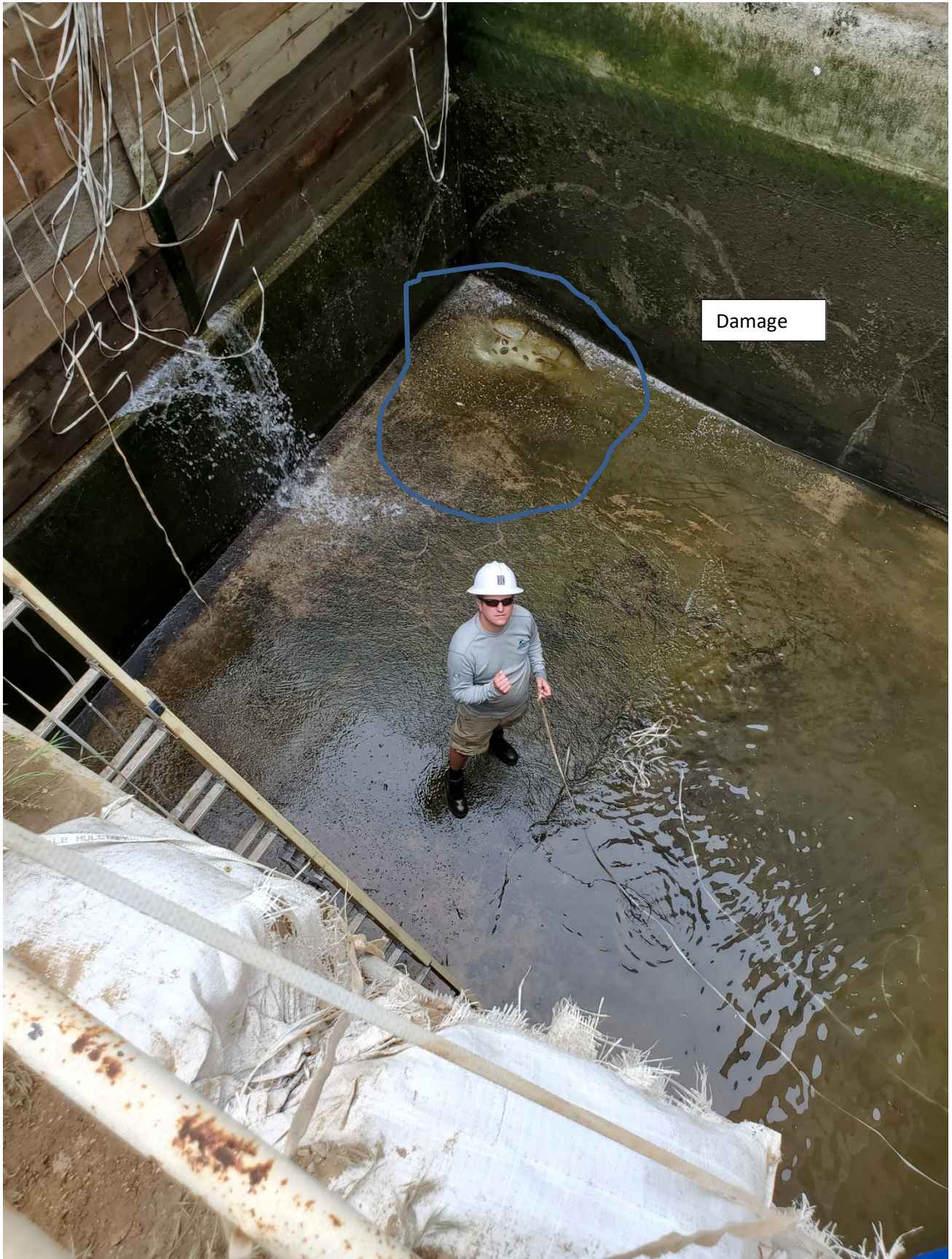
BAY 1 MOSTLY PUMPED OUT CONCRETE DAMAGE IN TOP CORNER
