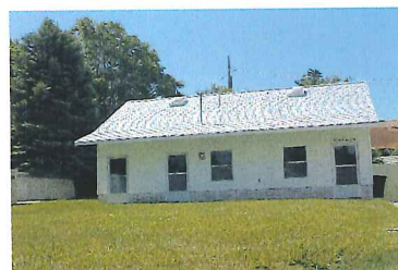
96 N 100 East (outbuilding)
