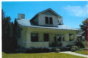
145 W Center Street B
