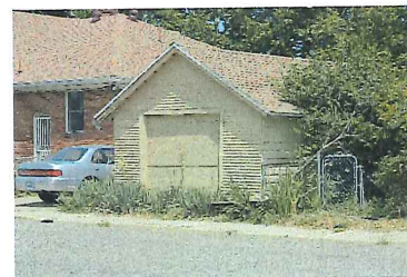
308 N 100 East (garage)
