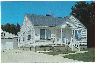
227 E Center Street C
