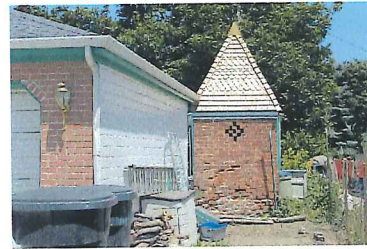
206 N 100 East (outbuilding)
