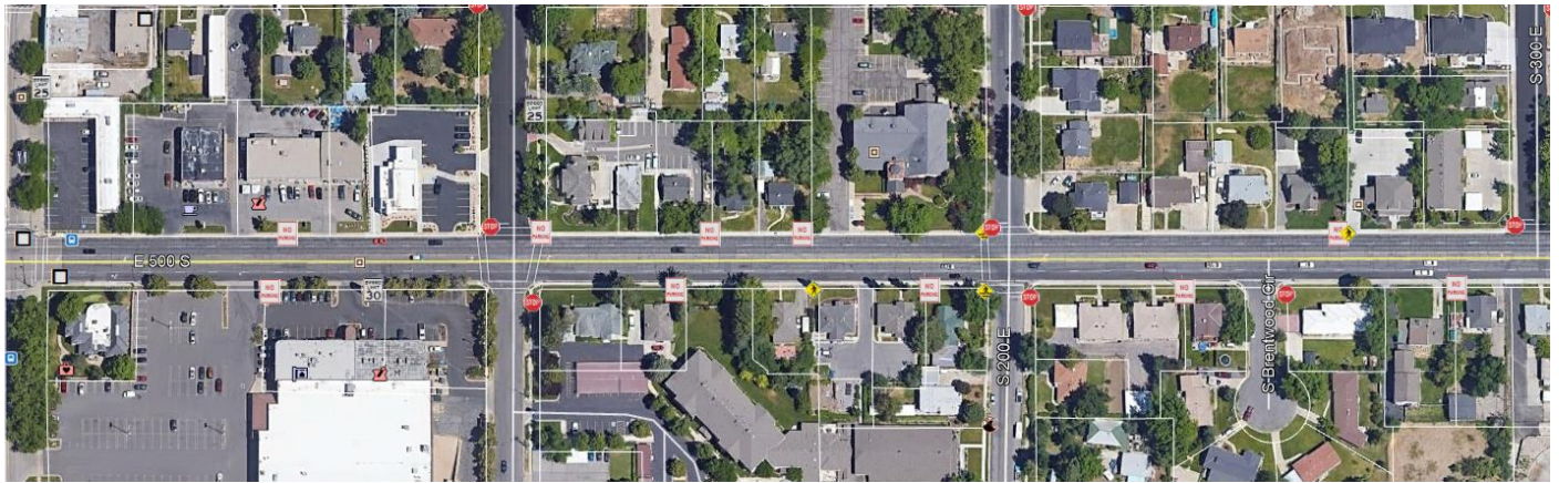
Figure 1 500 South Street, 100 E and 200 E intersections and existing crosswalk configurations, with existing signage.
