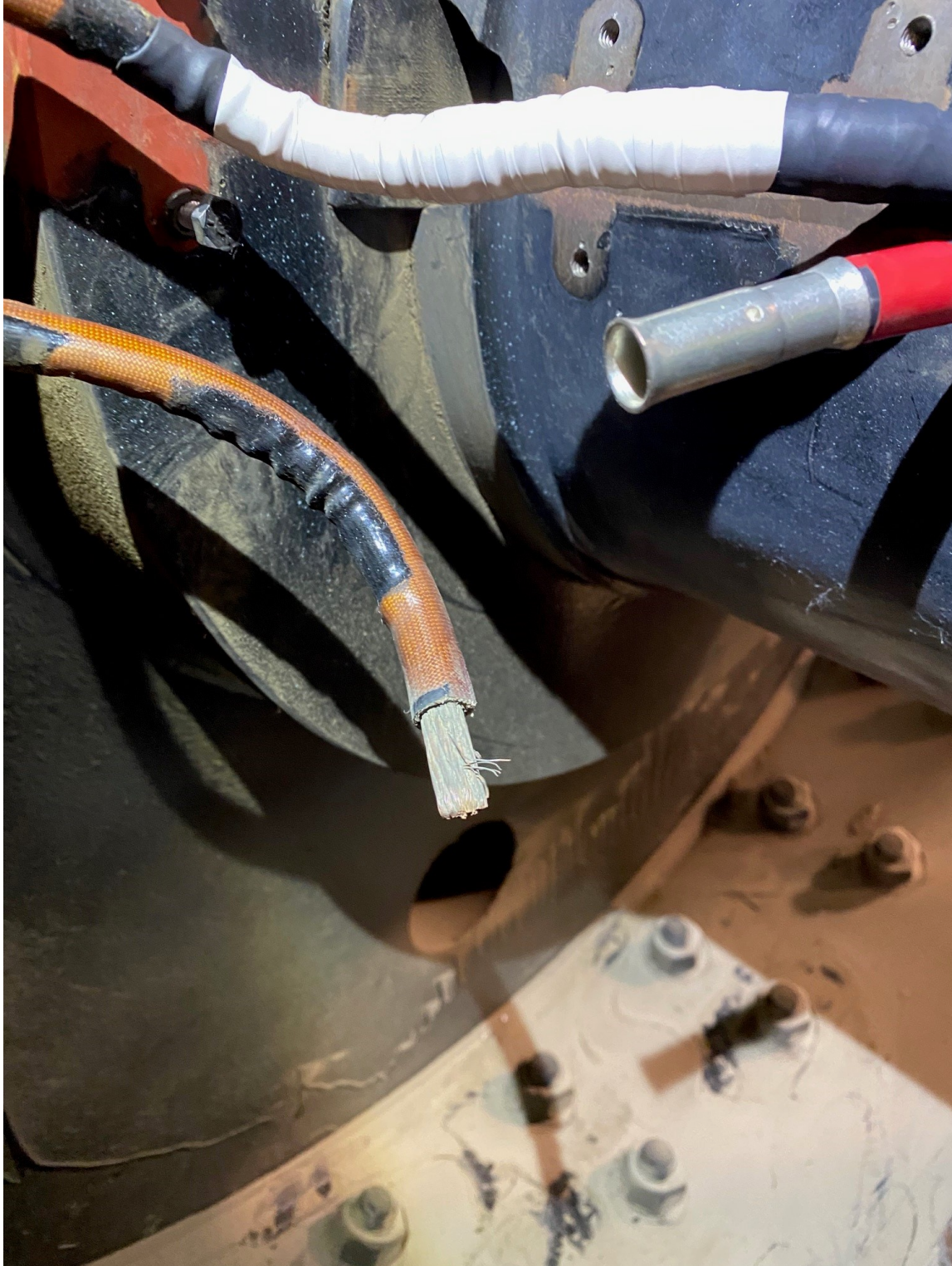
Temporary splice of new wire to old wire
