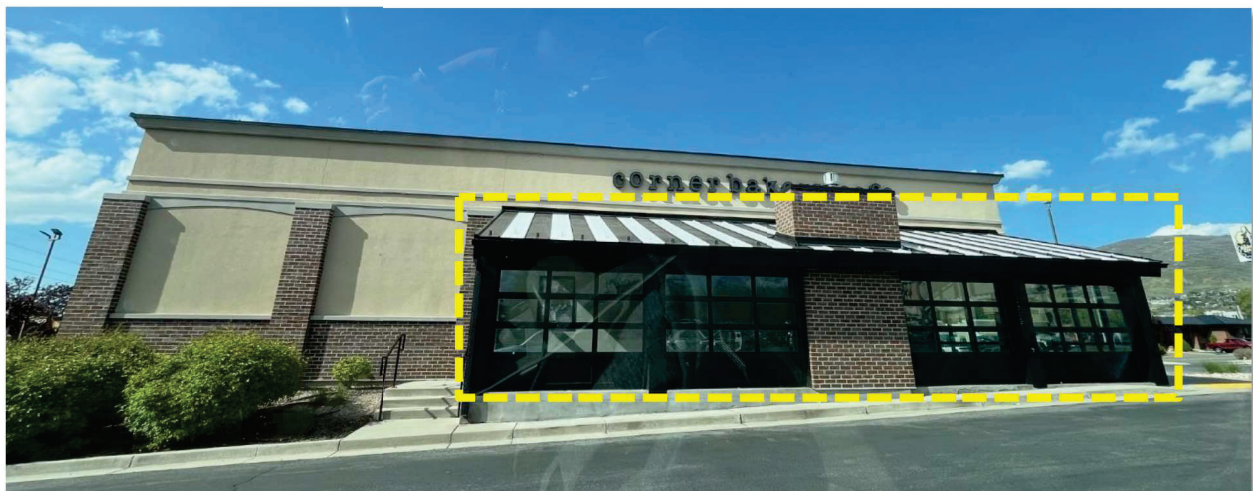
Image 1: Existing South Building Elevation – Photo Taken April 24, 2024
